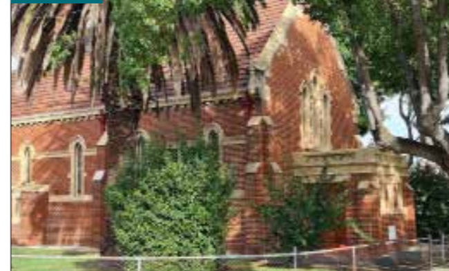
St Francis Xavier School and Church was built in 1935 and has strong ties to Aranmore College and Sacred Heart College. It is included on the Vincent Heritage List.
