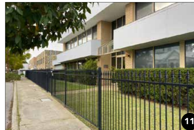
11 This fence is permeable, but the setback, tinted windows and landscape create a distance to the street.
