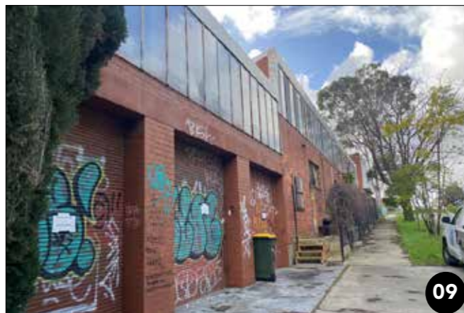
09 This existing warehouse offers no amenity or social surveillance to the public realm.
