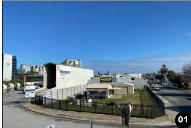
01 The concrete batching plants offer a future opportunity to revitalise Claisebrook.
