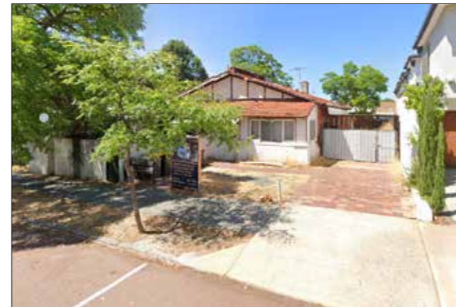
107 Summer Street Perth Draft Inventory
