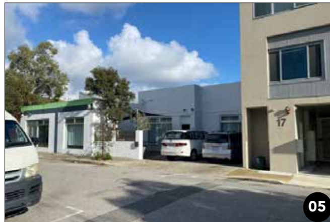
05 Gladstone Street is an eclectic array of buildings ranging from warehouses to new higher-density residential and pockets of lower-density character houses. The mix of heights and setbacks adds to the area's unique character.
