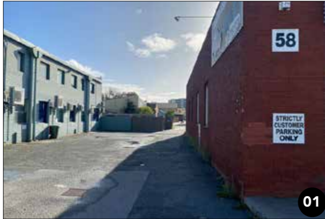
01 The built form along the laneway off Edward Street behind Lord Street offers limited activation. The lane is vehicle dominant.
