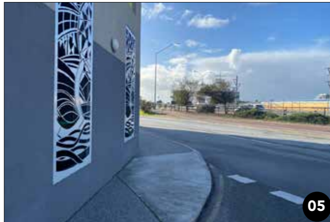
05 While parking on the ground floor offers passive surveillance, it feels like there is no activity, making the corner feel unsafe.
