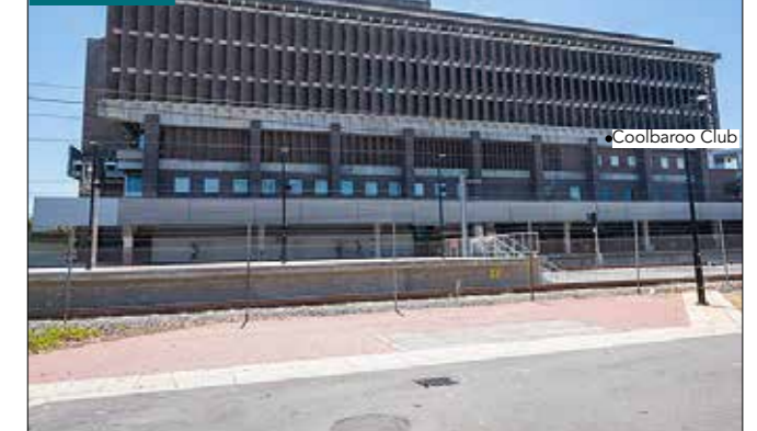
East Perth Terminal built in 1976 is a classic example of the brutalist style of architecture. It is included on the Vincent Heritage List and State Heritage List. Credit: Vanessa Pogorelic
