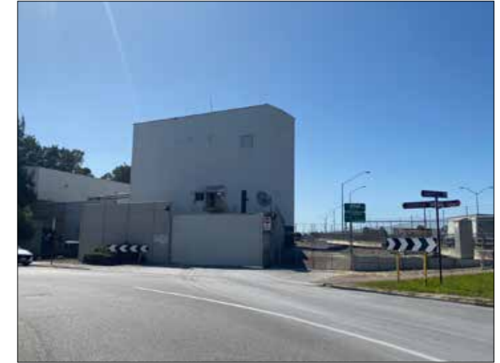
Existing concrete batching plant on Claisebrook Road.
