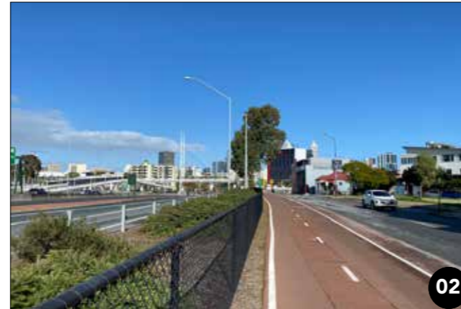
02 There is space for trees along the freeway as part of the green enhancement plan.
