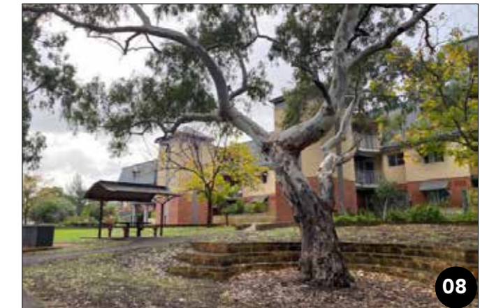
08 This four-storey residential building offers passive surveillance of this secluded park. The park feels like a private garden due to the surrounding built form.
