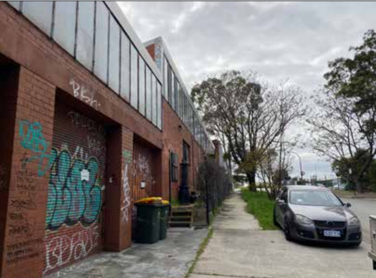
Pedestrian path needs rationalising.
