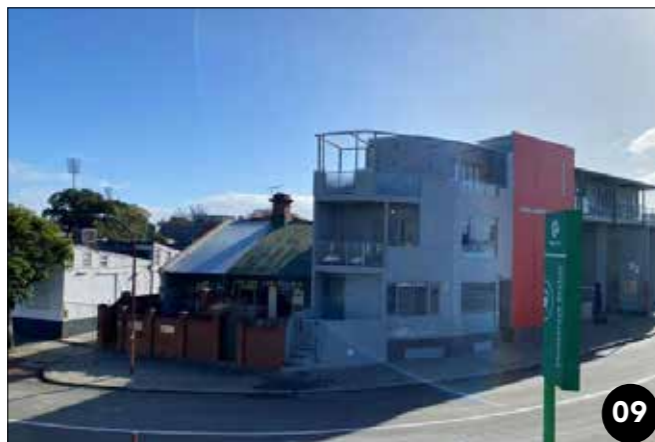
09 Examples of lower and higher-density residential sitting side-by-side differ in scale and materiality.
