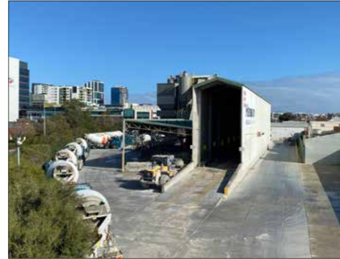
Existing concrete batching plant on Edward Street.
