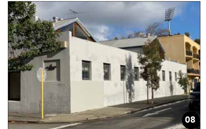
08 This residential warehouse conversion offers no social surveillance to the public realm.
