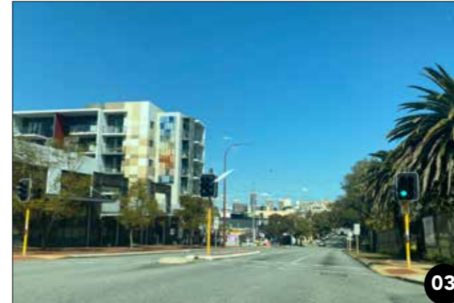
03 The higher-built form provides more housing opportunities, and the ground plane along Lord Street must have a human scale.
