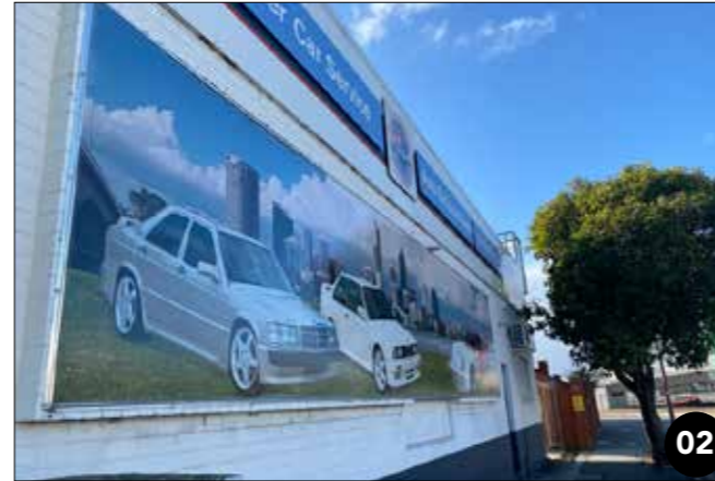
02 A blank billboard facade along Edward Street provides little to the public realm.
