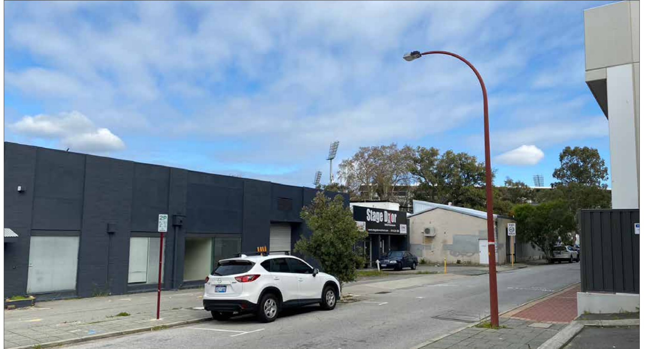
Concrete batching site to left as looking west down Caversham Street.
