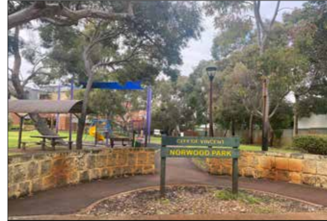
The limestone walled entry to Norwood Park creates a sense of arrival. The wall is approximately 700mm high, which is not comfortable for seating. The orange staining indicates the bore water has a high iron level.
