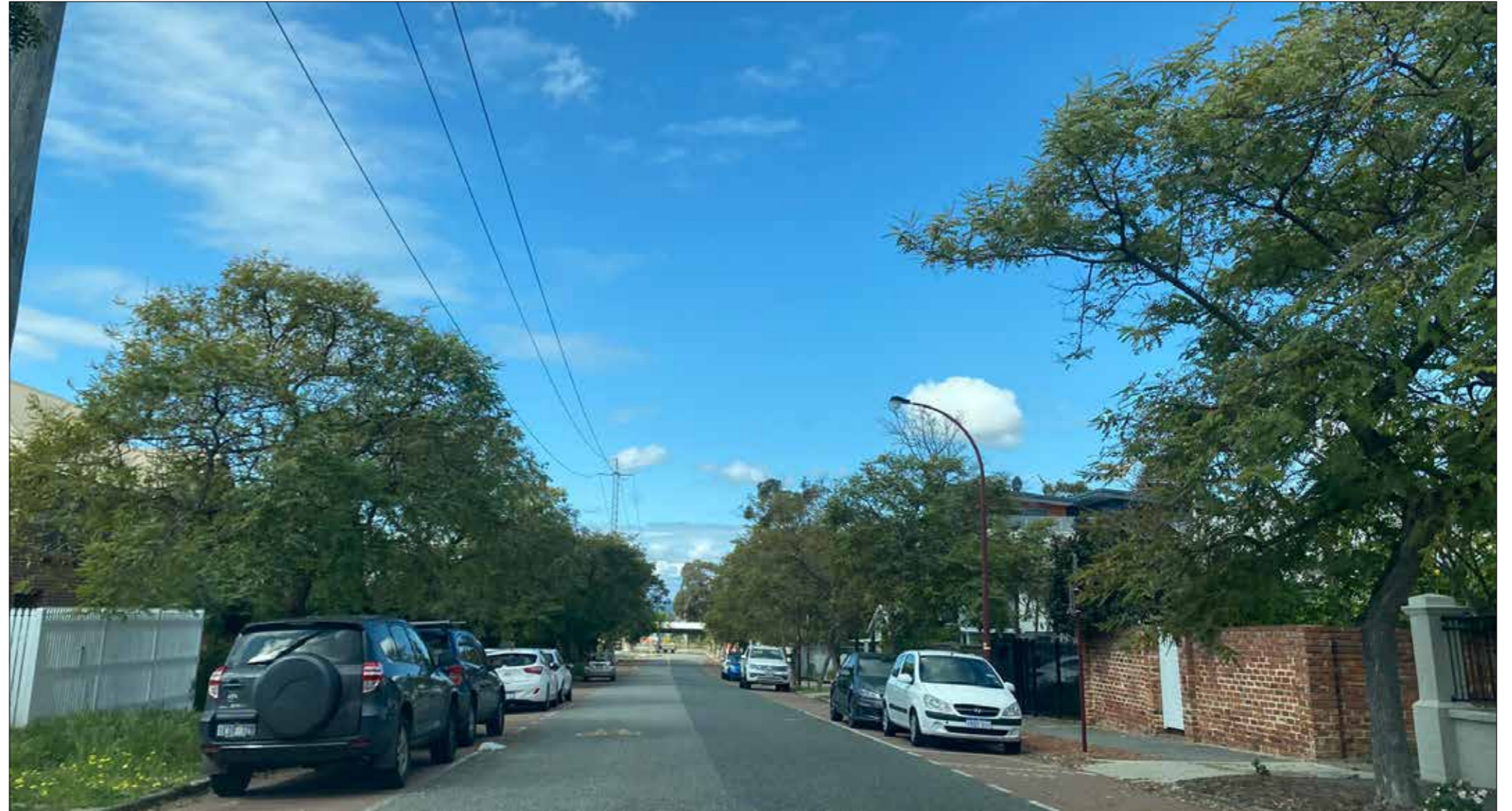
Summers Street is the only street with overhead power. Image is looking east down Summers Street towards East Perth Terminus.
