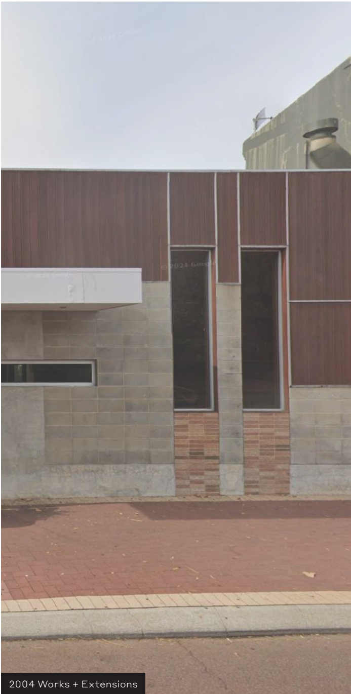
Concrete, masonry blocks, timber panelling, feature face bricks and chrome highlights, additional awnings added to entrances on Beaufort and Brisbane
