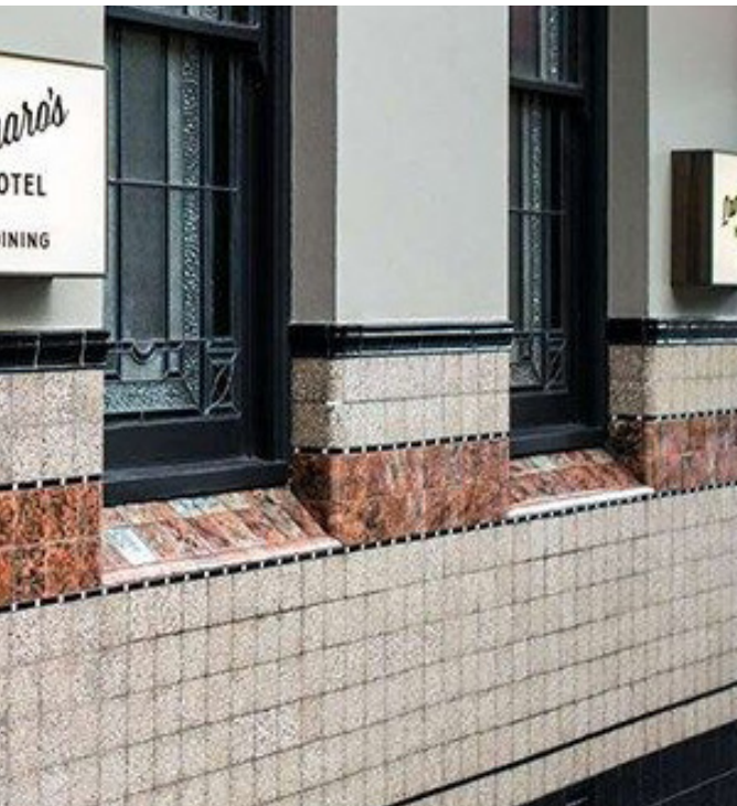
Restore, reinstate and repair the existing facade and fabric of the exterior.
