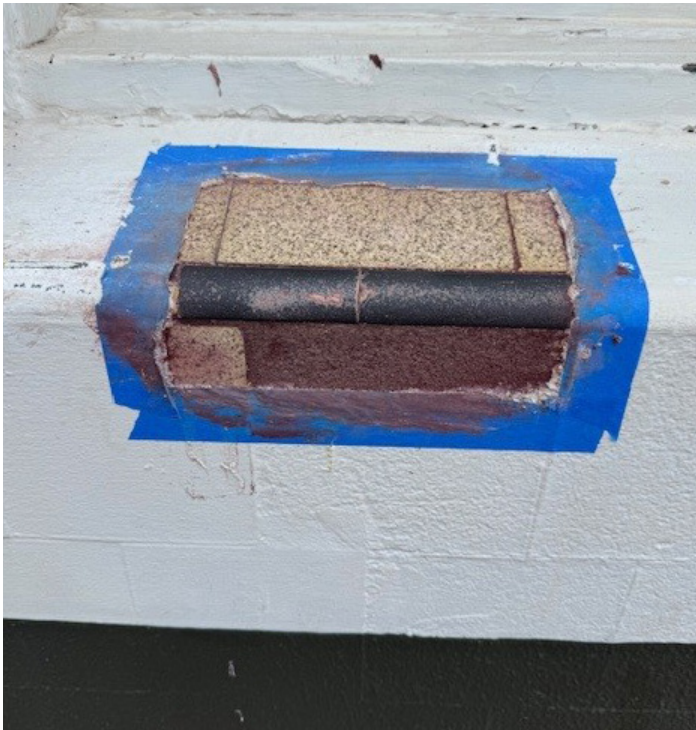
1930s tiling details to original windows
