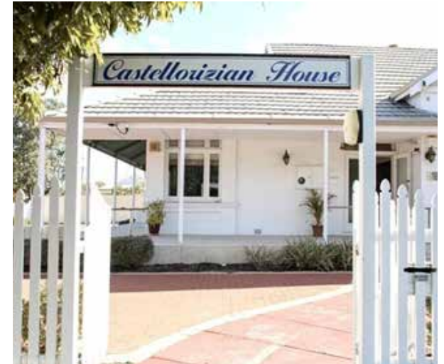
Castellorizian House, 160 Anzac Road 2020 (COV PHO6054)
