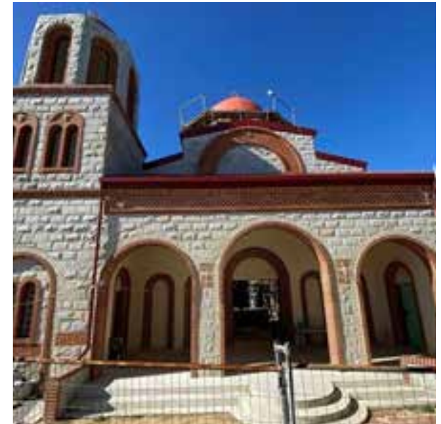
Macedonian Orthodox Church of St Nikola under construction, 2020 (COV PHO6073)
