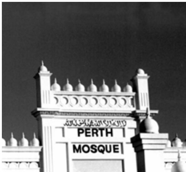
Parapet on the Perth Mosque 427-429 William Street Perth, c 2000 (COV PHO5877)
