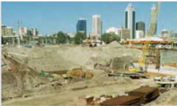
Northbridge Tunnel & Graeme Farmer Freeway under construction, 1997 Credit: State Library of Western Australia
