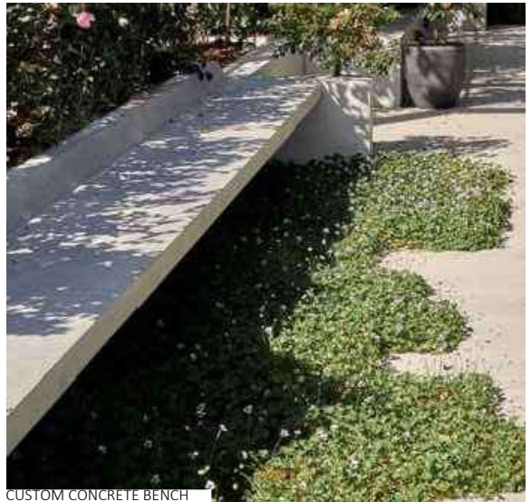
CUSTOM CONCRETE BENCH TO STREET LIBRARY CORNER
