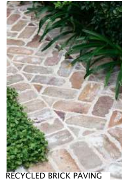
RECYCLED BRICK PAVING
