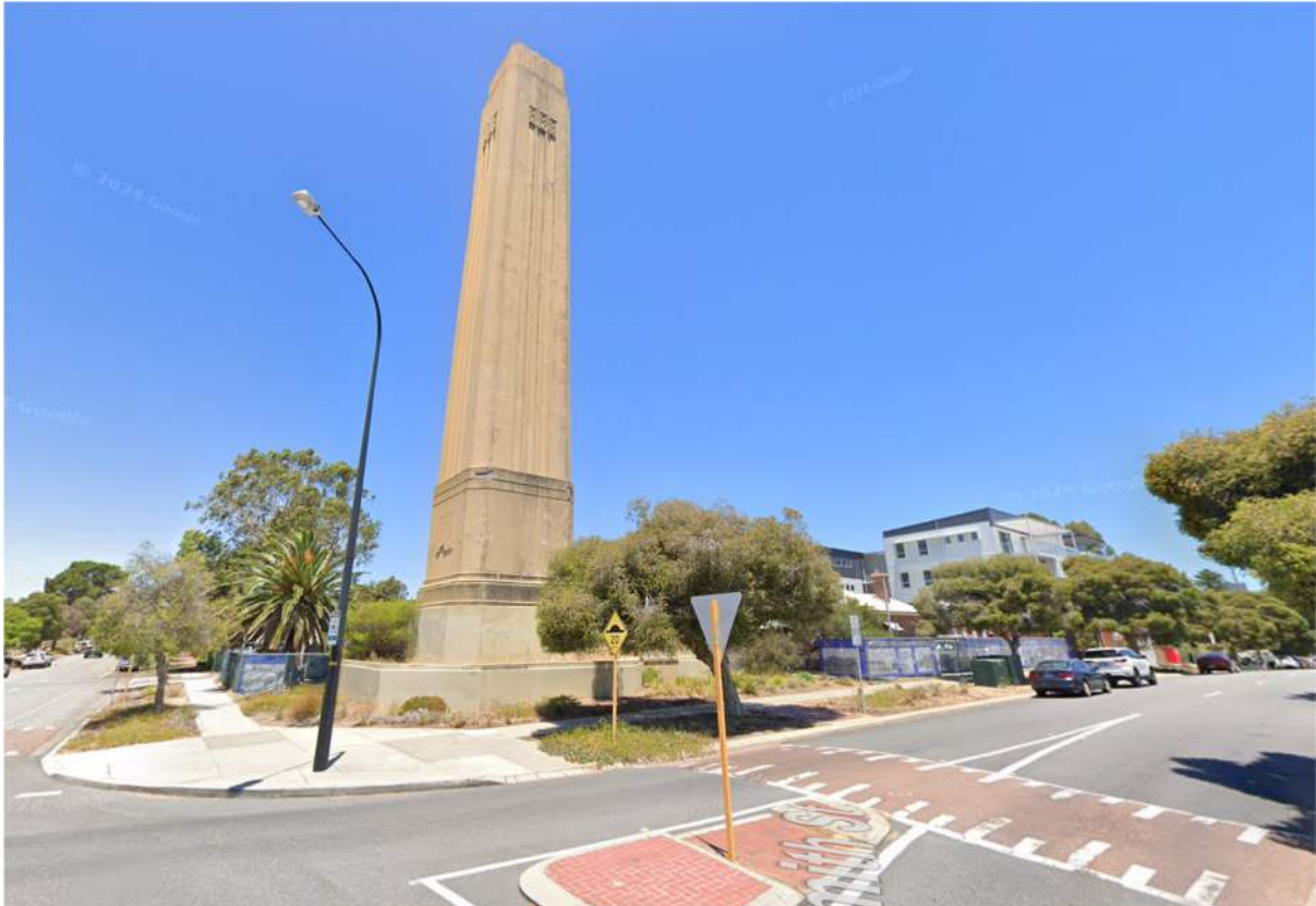
Photograph 6: Lincoln Street Ventilation Stack
