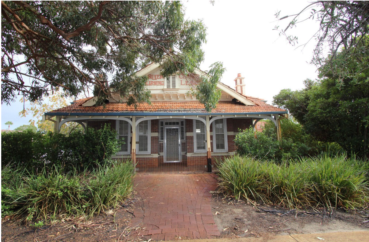
Figure 5 East façade of Silver Chain Nursing League Building will not be impacted by the Stage 1 development, but conservation work will assist in maintaining the place. Griffiths Architects March 2026
