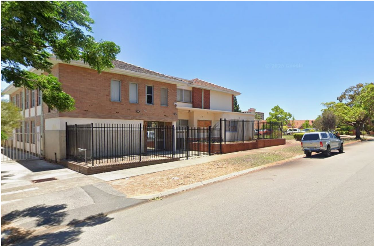
Figure 8 View from Wright Street, Northeast view of buildings to be removed and replaced. Google Streetview.
