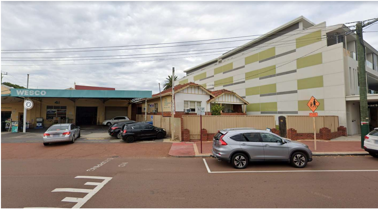
Photo 5: View of existing service station and residential dwelling adjacent to the four storey mixed use development on the neighbouring property, taken from Angove Street.
