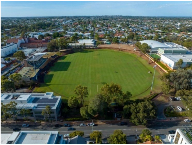
Figure 18: Aerial of Leederville Oval
