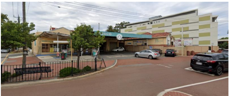
Figure 1: Street view of site
