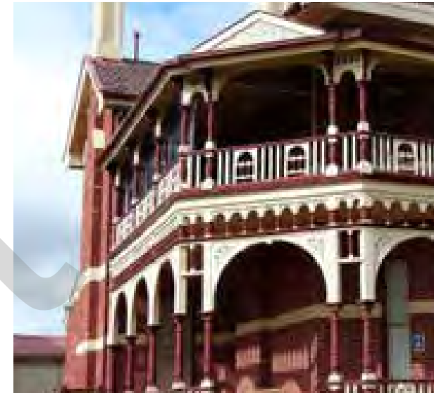
Dilhorn House at 2 Bulwer Street built in 1897 in Federation Queen Anne style (Heritage Place 02168)
