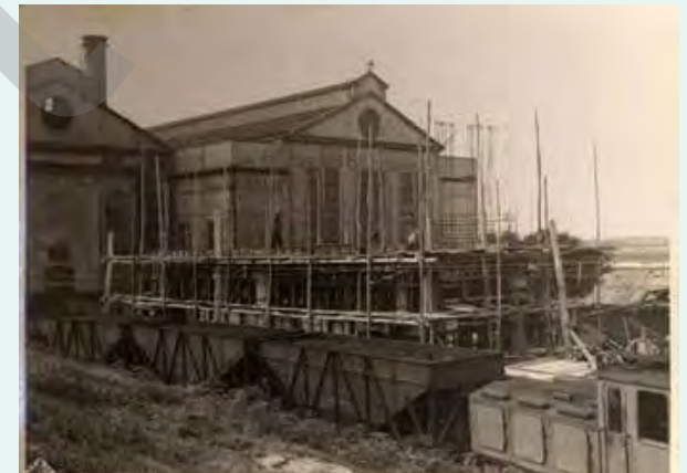
East Perth Power Station, 1936 (COV PHO1929)
