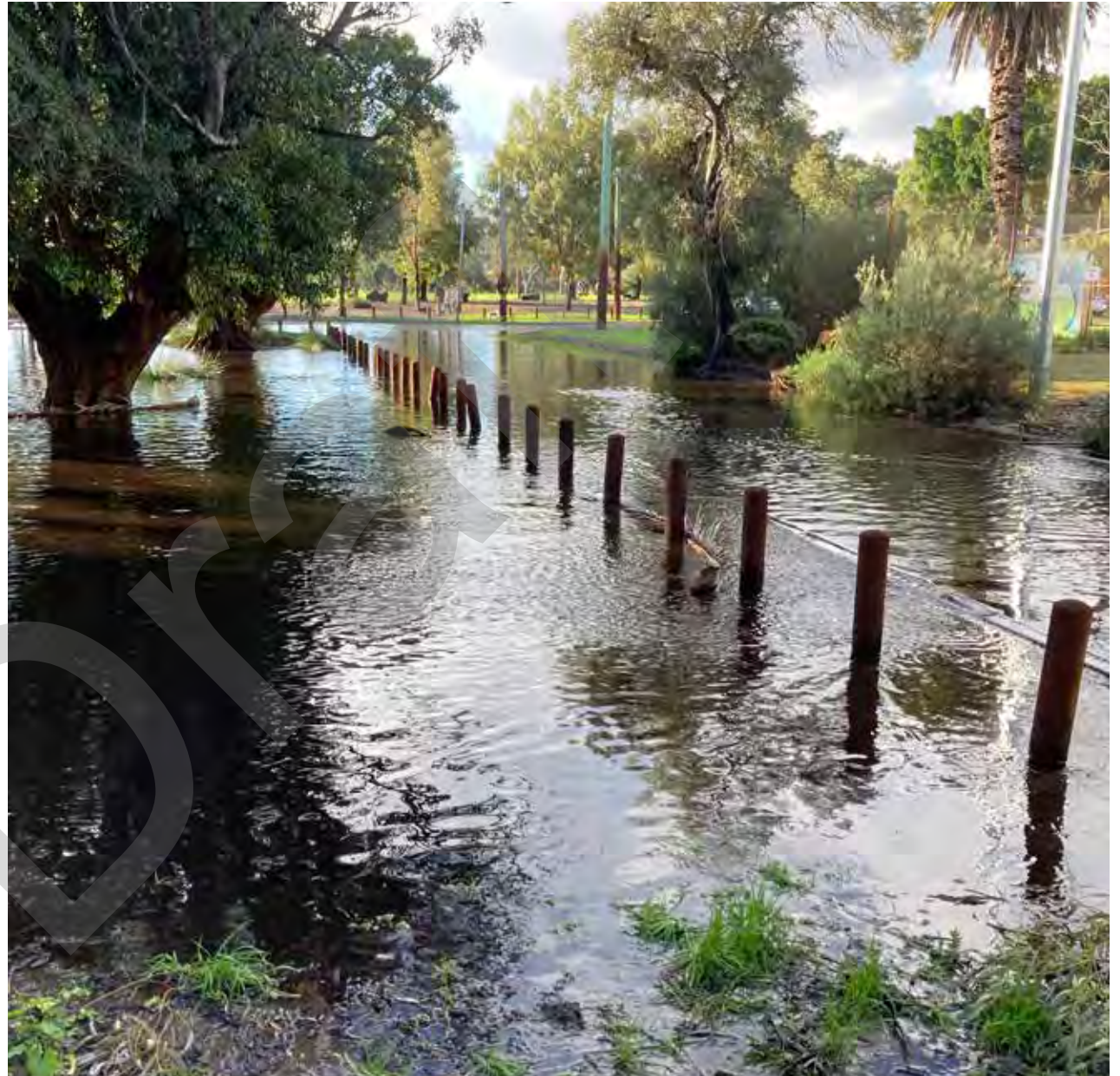
Flooding beside the Leederville Tennis Club, Britannia Reserve July 2021 (COV PHO6346).
