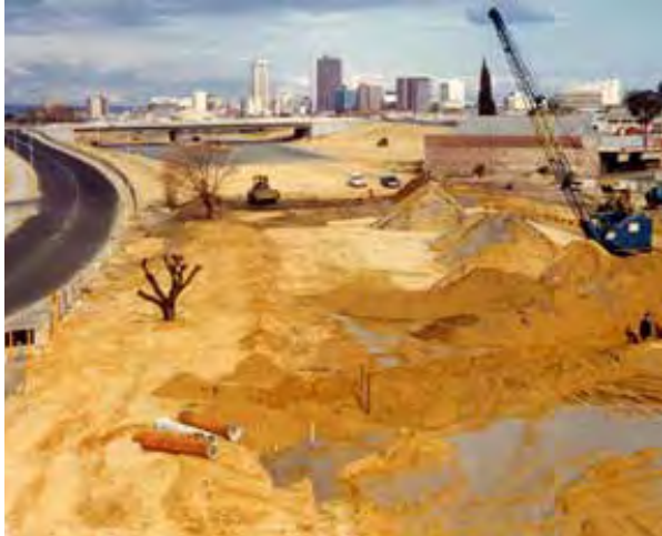
Construction of Mitchell Freeway extension at Leederville Parade, 1975 (COV PHO2577)
