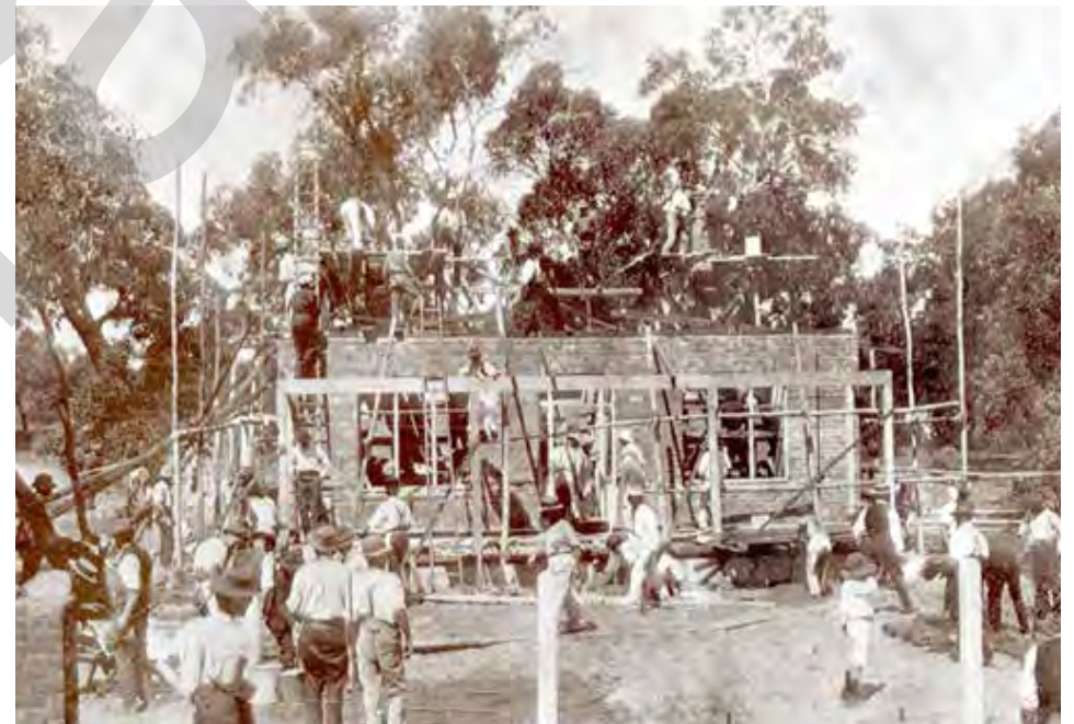
Volunteers at work constructing Anzac Cottage, 12 February 1916 (COV PHO1007)
